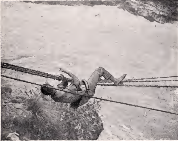
NATIVE CROSSING ROPE BRIDGE
